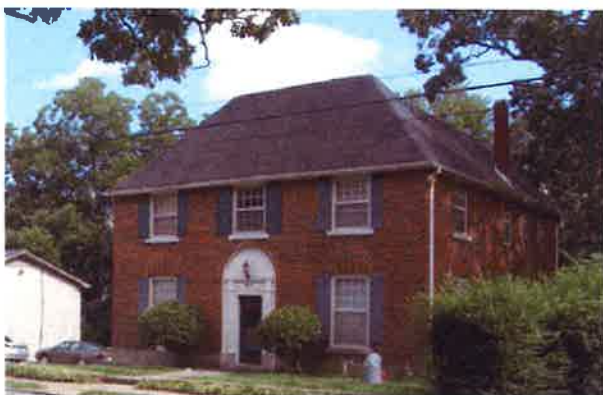
FOUR APARTMENT/MANSION BUILDING, HILLCREST
